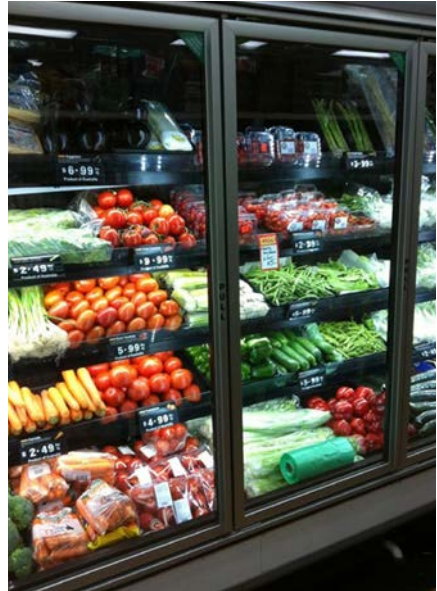
Retrofit glass doors fitted to 5-year-old Austral open-front merchandisers at Foodworks in Graceville Queensland 42
