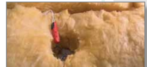
Clearance of 50mm around downlight
