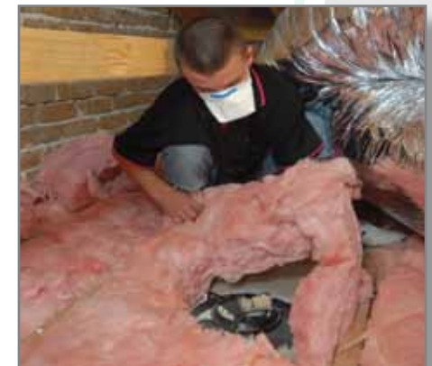
Clearance of 50mm around downlight
