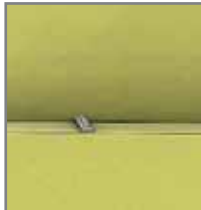
Electrical cable running between layers of thermal insulation
