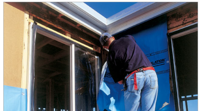
Installing wall insulation.
